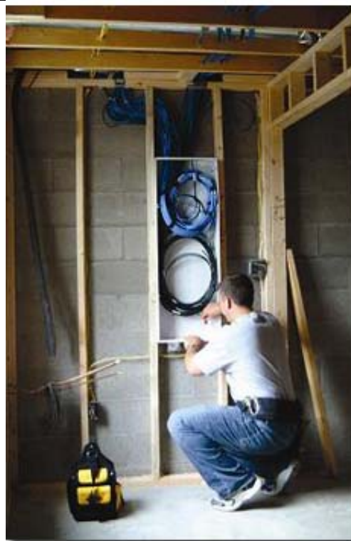
Electronic Systems Contractor installing structured wiring.
